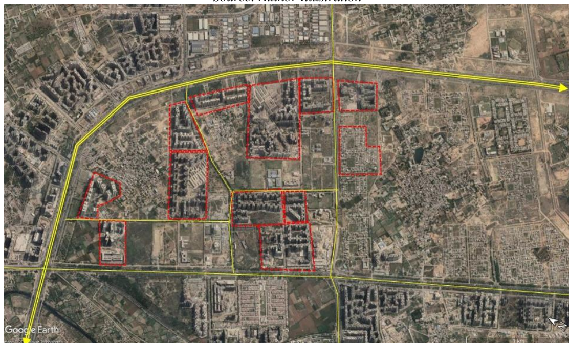
Figure 15: Satellite image of G. NOIDA with illustration highlighting the regular plots and road networks Source: Author Illustration
