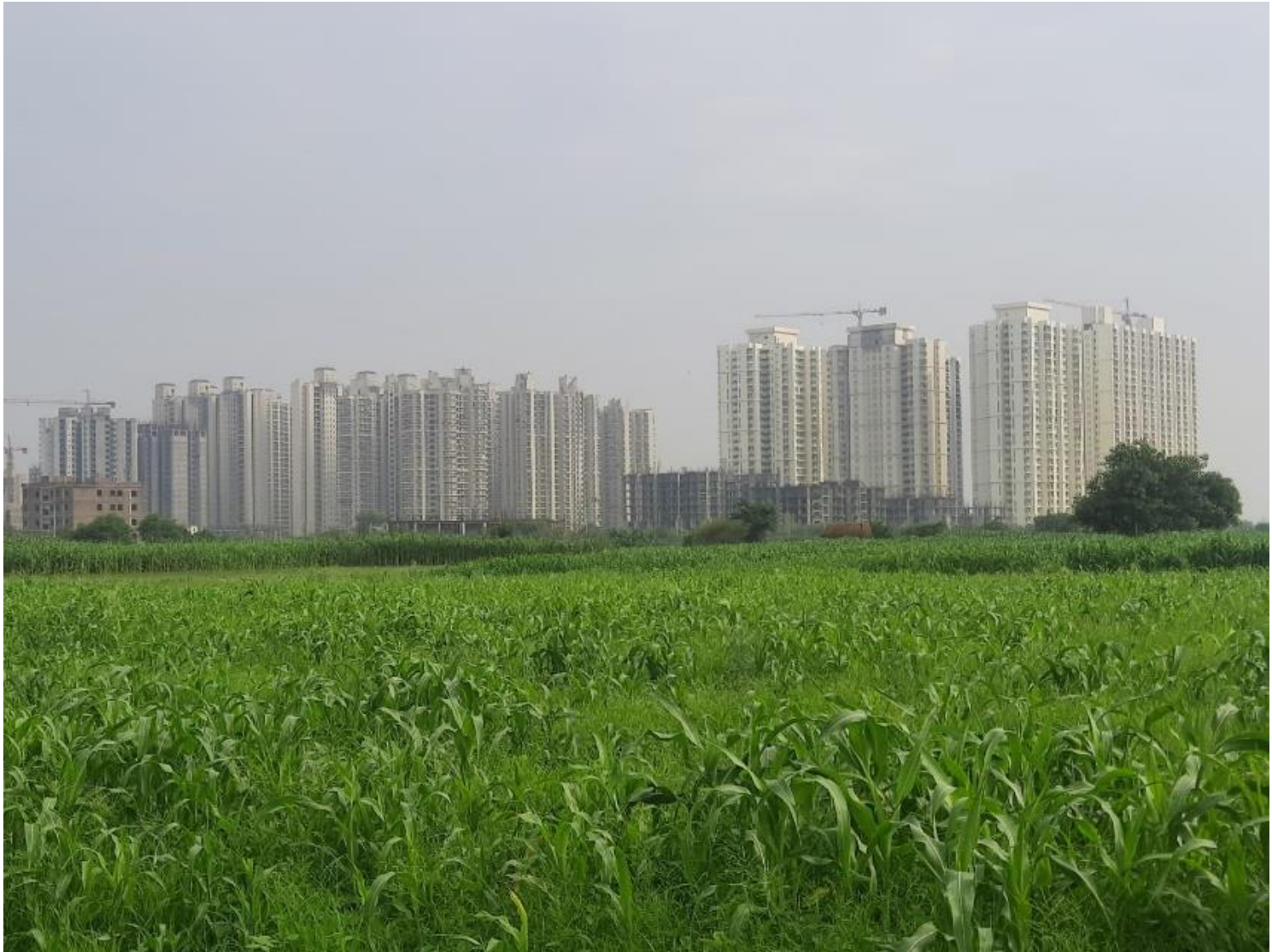
Under construction Project in Greater Noida, India in close proximity to agricultural land
