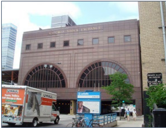
Chicago Stock Exchange over Congress Parkway. Source: Will's Photostream cited from https://www.chipublic.org/blogs/post/technology-that-changed-chicago-air-rights/
